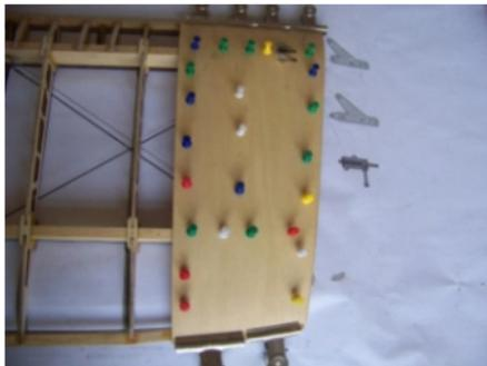
(13) Glue 1mm plywood board (up and down).
